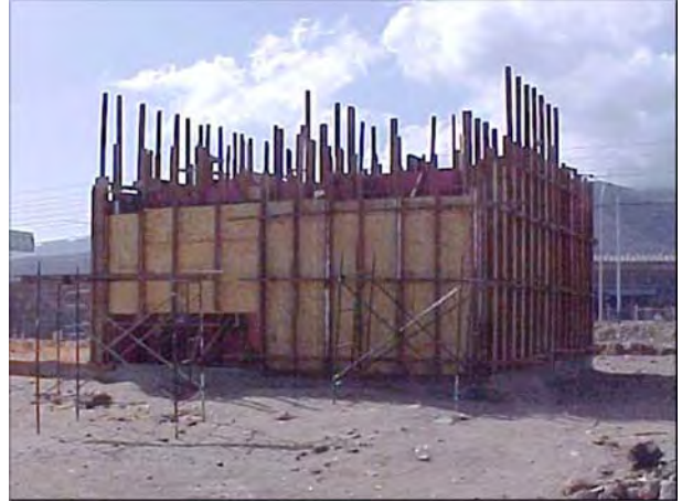
IN-SITU CAST OR CAST-IN PLACE
