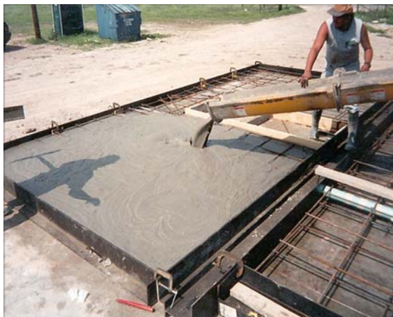
LITEBUILT® AERATED LIGHTWEIGHT PANEL CASTING
