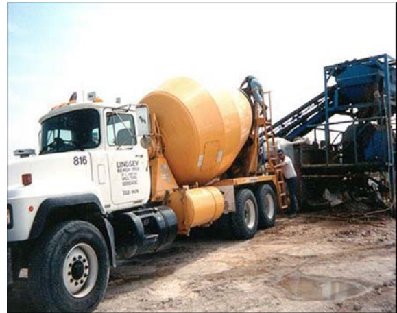
LITEBUILT® FOAM BEING INJECTED INTO CONCRETE TRUCK
