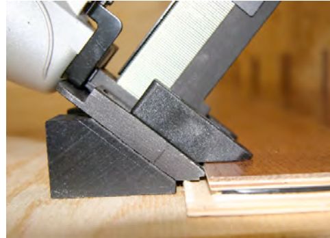
Fig. 14 – Staple gun correctly positioned
