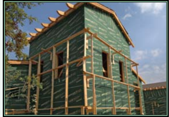
StructGuard ® TS can be fastened using nails, screws or staples and adds a measure of fire and mold resistance other sheathing alternatives can't match.
